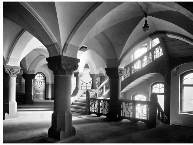
Fig. 6. Main Edifice of Construction Crafts School and Higher School of Machine Building. The hall interior with the main staircase on the second floor in circa 1904 (photo: E. van Delden, H. Götz. [University Library 'Na Piasku' in Wrocław, Graphic Collections Department (OZGBU), File No 1170])
