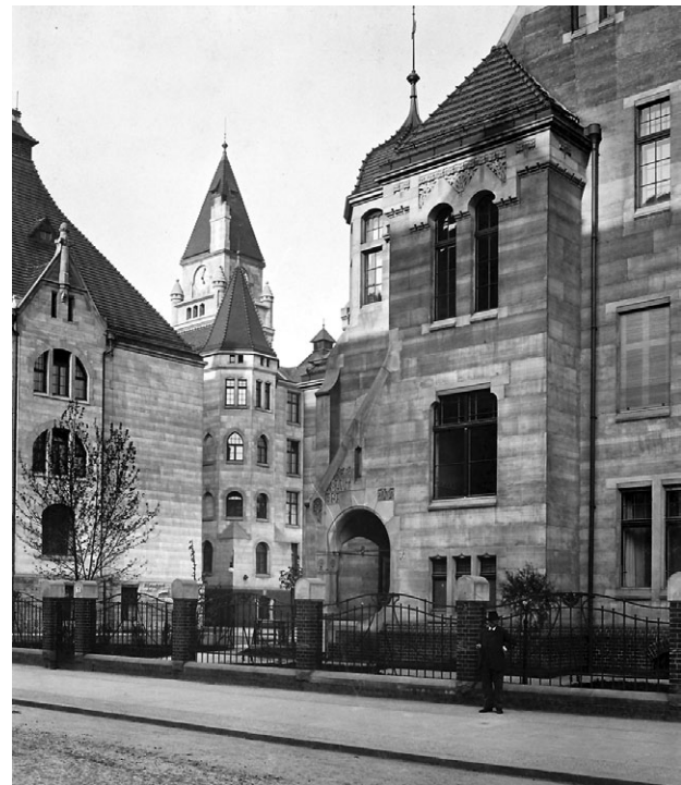
Fig. 4. View of the main building fragment and residential house of the school from the south-western side in circa 1904 (photo: E. van Delden, H. Götz [University Library ‘Na Piasku’ in Wrocław, Graphic Collections Department (OZGBU), File No 1167])
