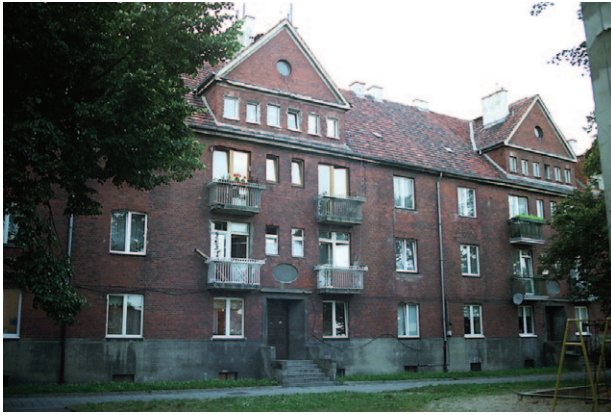
Fig. 7. Wrocław, the building of the J. Gotthelf Foundation, rear elevation, photo 2005
