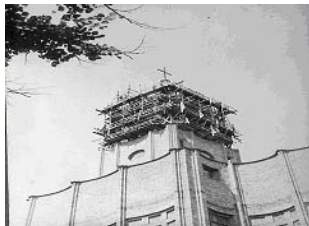
Fig. 6 Building of the reinforced concrete tower top [1]
