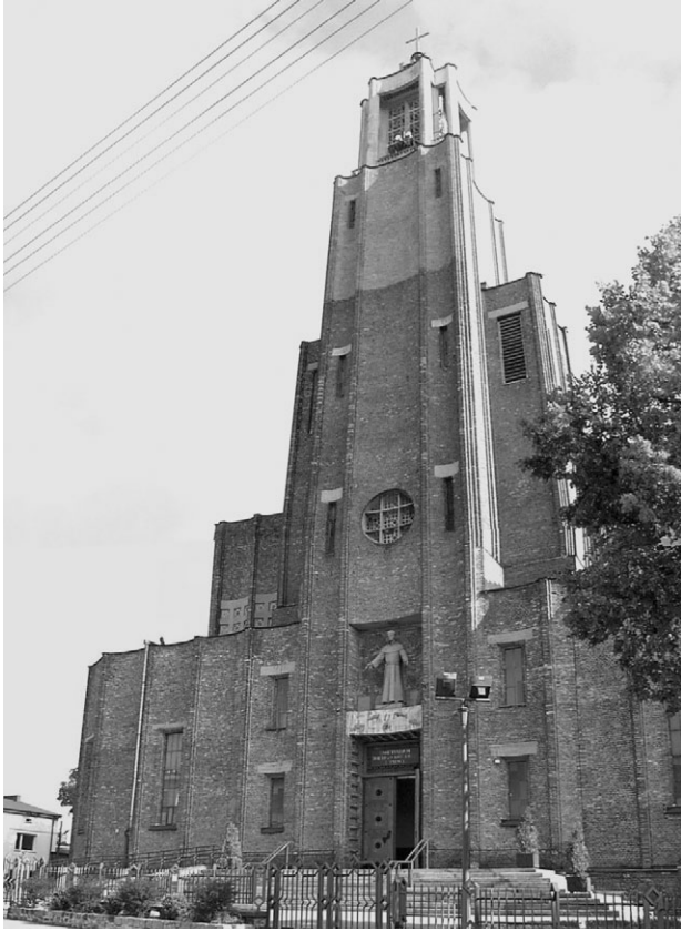
Fig. 12. St. Anthony's Church – front façade, existing state [2]
