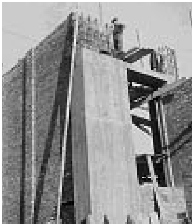
Fig. 2. Building church walls, in the foreground we can see a reinforced concrete column [1]
