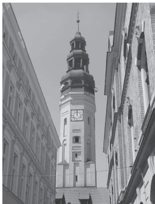
Fig. 2. View of the town hall from the south-west (photo: A. Legendziewicz) Il. 2. Widok wieży ratusza od wschodu (fot. A. Legendziewicz)
