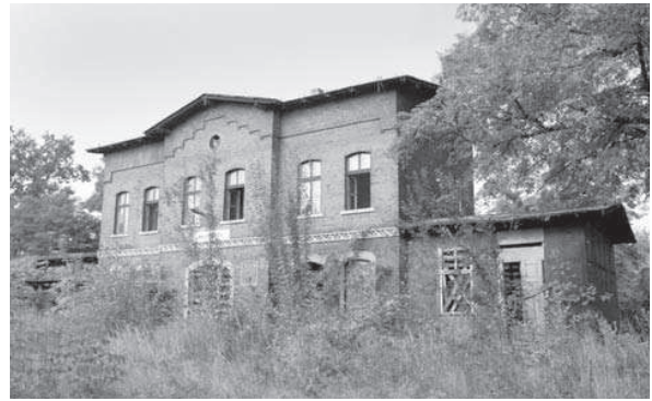
Fig. 7. Biała Prudnicka station. The station is abandoned and squalid. In comparison with other stations on this line it boasts richer brick details (photo: M. Konopka, 2009)
