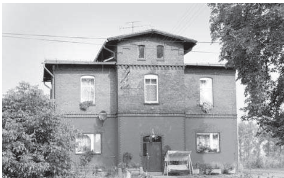
Fig. 2. Lubrza station. The building has been transformed into living quarters. Windows on the ground floor have been rebuilt and all the frames have been ineptly exchanged. The ground floor elevation has been painted (photo: M. Konopka, 2009)
