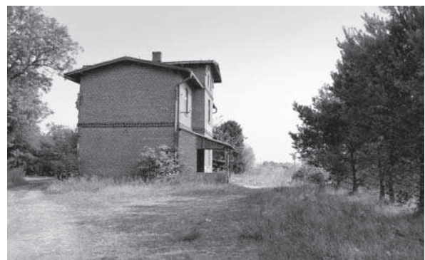
Fig. 9. Strzelczki station. The building is abandoned and unsecured, and the area around squalid (photo: M. Konopka, 2009)
