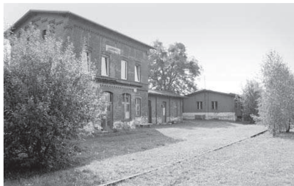
Fig. 3. Krapkowice station. The building is inhabited on the first floor. The ground floor has been unused since 1990. The building is squalid. New and ill-selected window frames in the flat are explicit (photo: M. Konopka, 2009)
