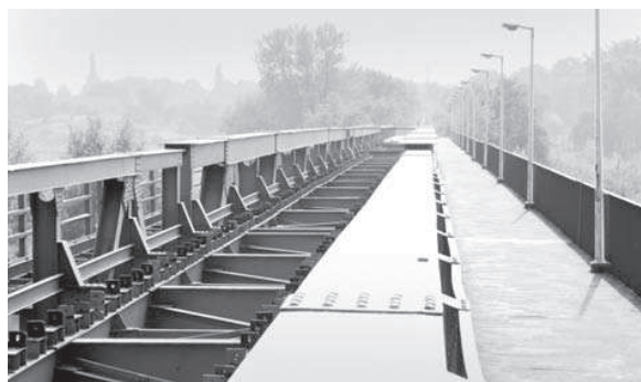
Fig. 5. The pedestrian footbridge on the railway bridge over the Odra between Krapkowice and Otmęt. The track was removed after the July 1997 flood. A pedestrian footbridge has been in operation here since the 1930s. At present the reconstruction of the bridge into a road one is under consideration (photo: M. Konopka, 2009)
