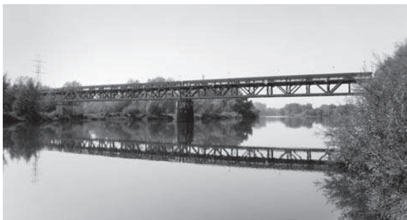
Fig. 4. The railway bridge over the Odra between Krapkowice and Otmęt. The western span fell down during the July 1997 flood. It was repaired but the traffic has not been restored (photo: M. Konopka, 2009)
