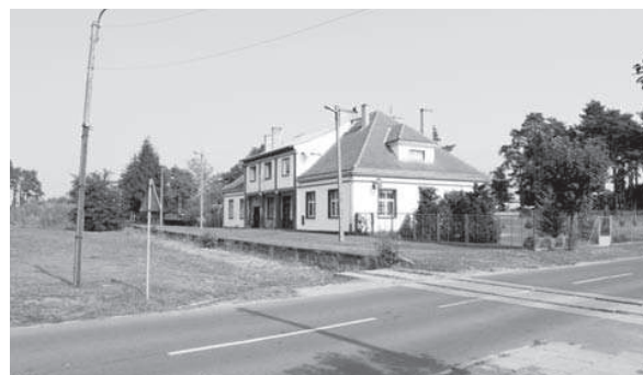
Fig. 1. Krapkowice Otmęt passenger stop. In the foreground the hole after a removed track. The railway station building has been completely transformed into living quarters and is preserved in good condition. It is one of the few modernist stations in the Opole region (photo: M. Konopka, 2009)
