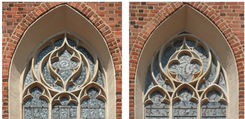
East windows of the south façades
