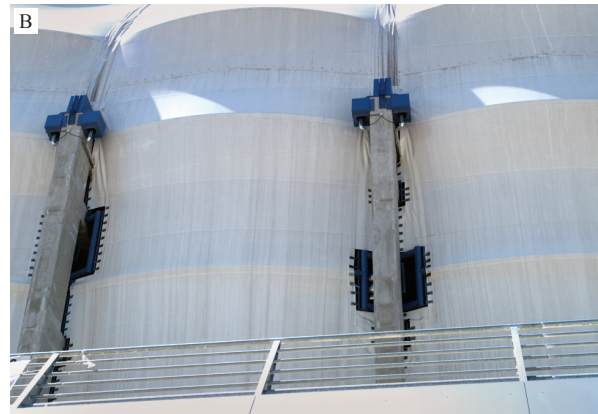
Fig. 6A & 6B. Photos of the façade of the stadium in Poznań. The photo A shows the rhythm of the supporting columns and hopper heads. Below a visible network roofed platform for protection against snow. The photo B shows the rainwater runs. In this case the designer did not design a gutter going along the lower edge, allowing it to drop freely from the edge (photo: M. Pelczarski)
