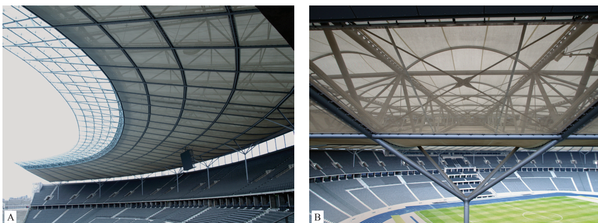
Fig. 5A & 5B. Photo (left) of the interior of the stadium in Berlin. Visible membrane stretched under the roof is an architectural cover increasing the beauty of the interior as well as acoustic barrier (photo: M. Pelczarski).
