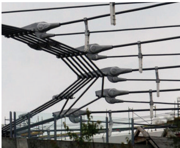
Fig. 9A. View of two clamps which broke while raising the cabling. Photo: Dawid WhiskeySix – forum gkw24
