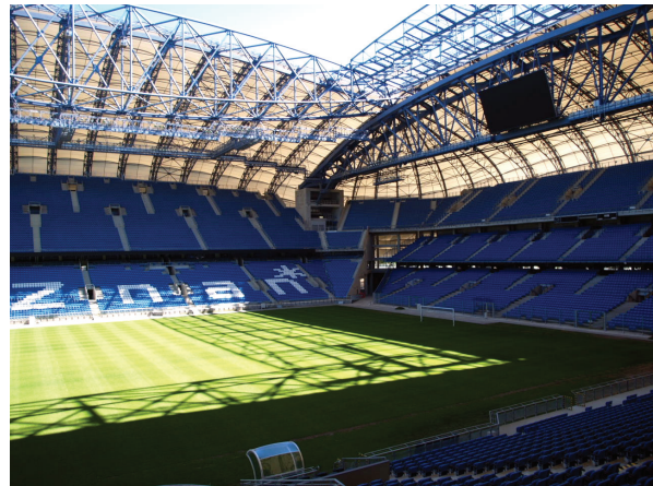
Fig. 3A. Photo of the interior of the stadium in Poznań and the view of the primary 160m long truss with the secondary 135m long, elliptical truss supported on it. The photo shows the “optical ballast” suspended above the heads of thousands of viewers (photo: M. Pelczarski)
