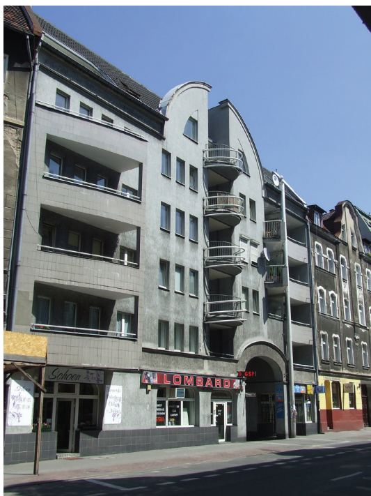
Fig. 4. An in-fill residential building at Poznańska Street 34, 36, 36a in Poznań dating back to the 1990s by Klimaszewska & Biedak, an architects. View from the street (photo by A. Nadolny, 2011)
