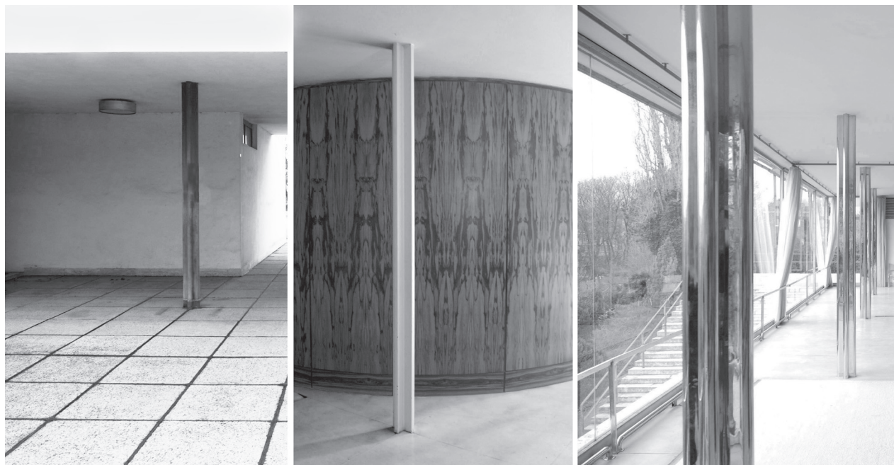
Fig. 7. The three types of columns in Villa Tugendhat (photo by A. Cervilla García, December 2009)
