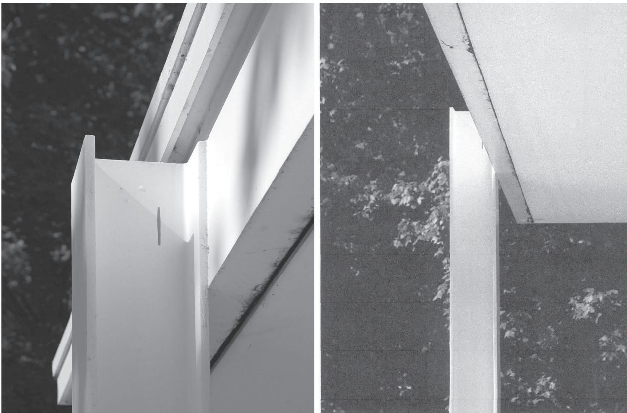
Fig. 13. The tangent union between column and beam in Farnsworth House (photo by A. Cervilla García, September 2012)
