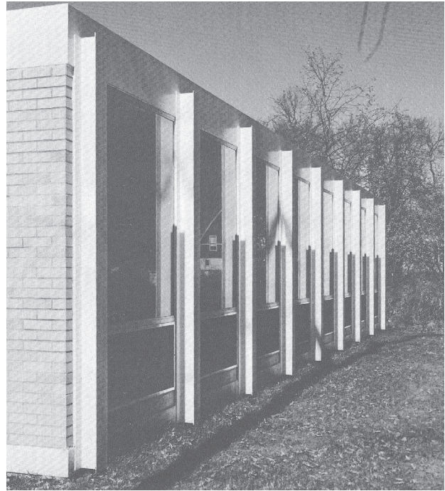
Fig. 14. Steel cage-type facade, in which Mies multiplies the number of columns (Hedrich-Blessing [10, p. 178])
