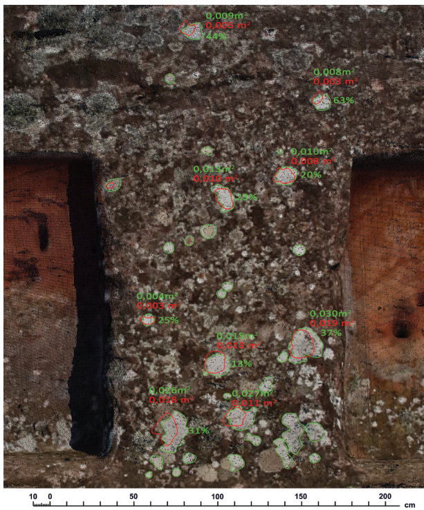
Fig. 9. Wall with niches from sector S08. Orthoimage from the 3D point cloud obtained in 2016 with information on lichen spread in 2006 (red colour) and 2016 (green colour) (elaborated by A. Kubicka)
