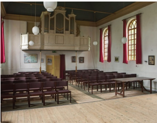
Fig. 4. View of the interior of the former church in Klein Wetsinge towards the porch. Condition before renovation, 2011 (source: [20])
