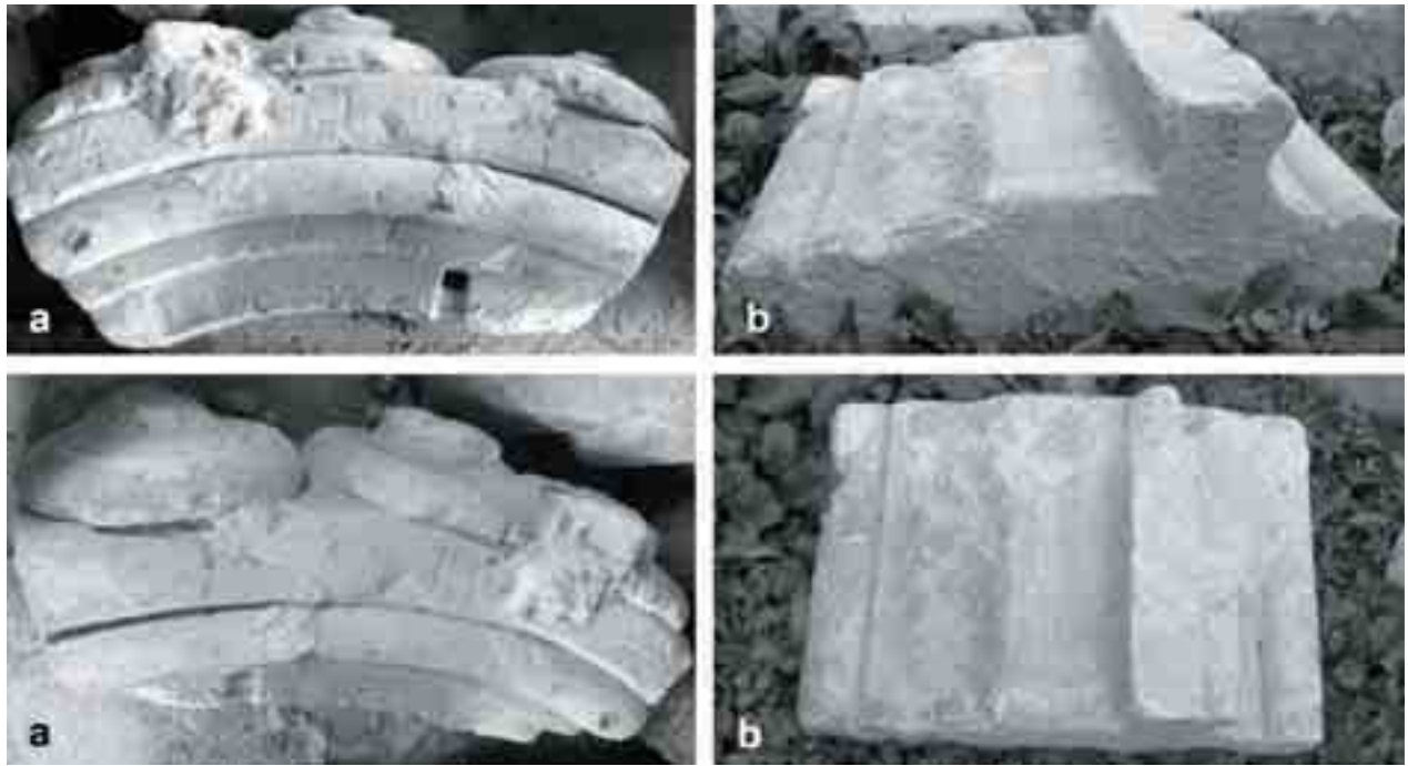
Fig. 6. The fragments of the rose window found in September 2005: a) the hub of the rose window b) the outer frame of the window
