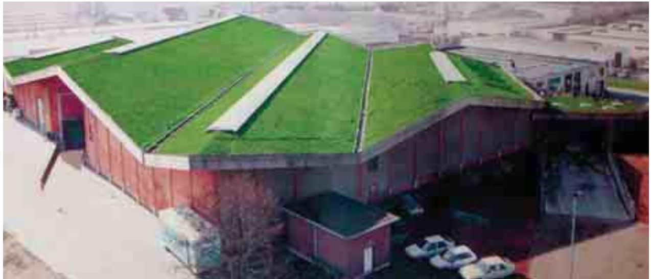
Fig. 6. General view of Ecover factory in Oostmalle. The picture shows grass on the roof which was later exchanged for sedum
