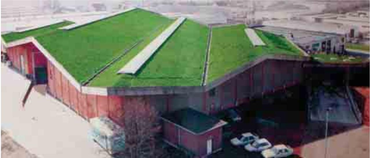
Fig. 6. General view of Ecover factory in Oostmalle. The picture shows grass on the roof which was later exchanged for sedum (photo: archive of Mark Depreeuw)
