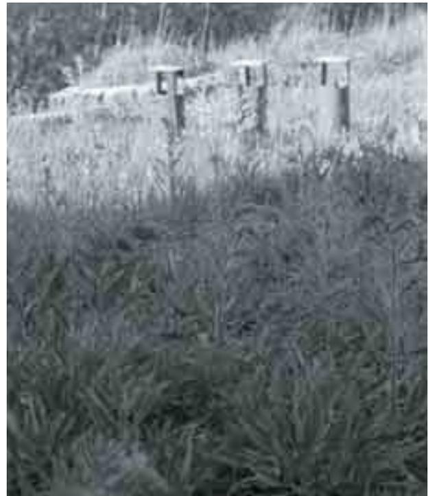
Fig. 2. Various vegetation on a brownroof over staff facilities building in syenite mine in Niemcza, Poland. The picture is taken a year after the soil from the surroundings was elevated onto the roof. No vegetation was planted (photo: M. Baborska-Naróźny)
