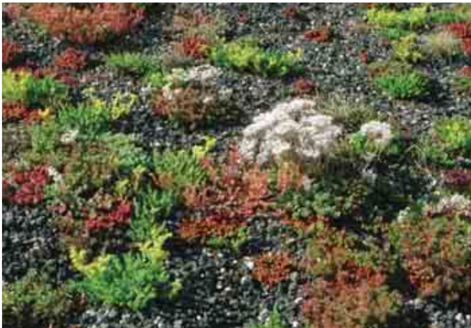
Fig. 1. Sedum cover on extensive roof one year after planting
