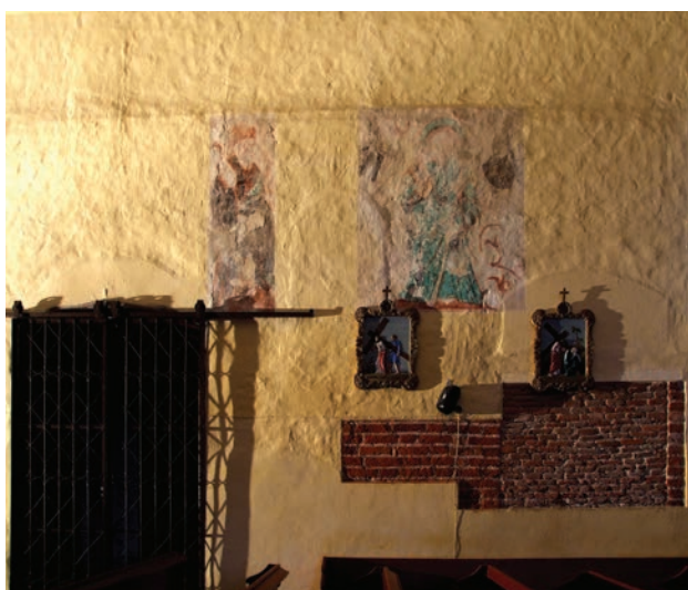
Fig. 2. Photograph of the inner face of the wall in raking light, a base for further analysis (detail of the south wall) (photo: J.M. Arszyńska)
