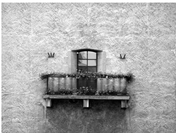
Fig. 5. Balcony of the town hall tower (photo: J. Salm)
