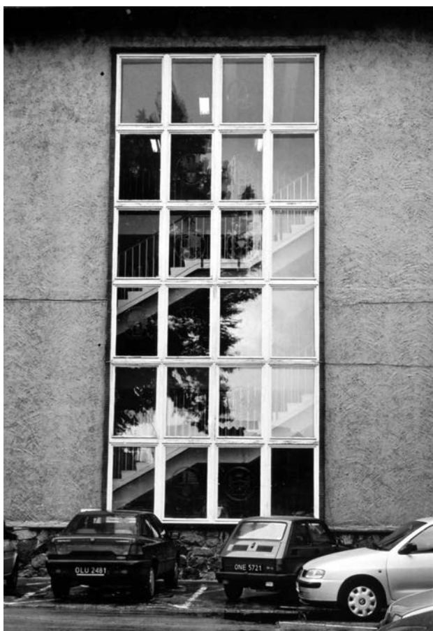
Fig. 9. Staircase glasswork (photo: J. Dobesz)
