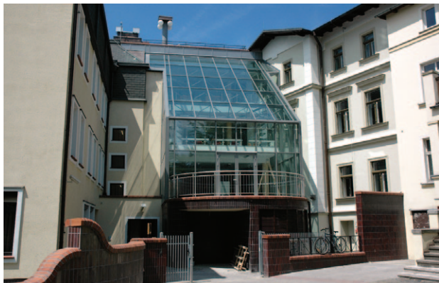
Fig. 3. View of Książnica Karkonoska at the side of block interior. A new glassed-in part connects other structures: secessionist tenement house (on the right) and the building from the 1990s (on the left) (photo: P. Amałowicz).
