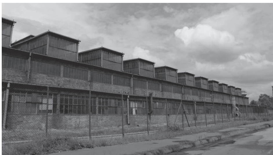
Fig. 13. Stalowa Wola, industrial halls of Metal Factory in the steel frame construction system. Photo by author, 2010
