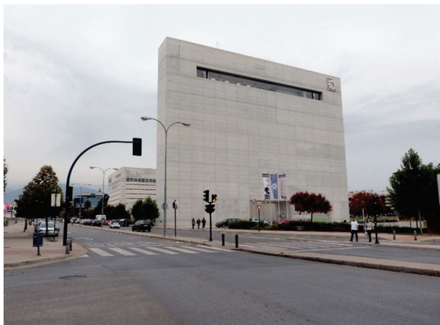
Fig. 3. Architectural complex (Cube & Museum, in the foreground) (photo by F.A. García Pérez, 2016)
