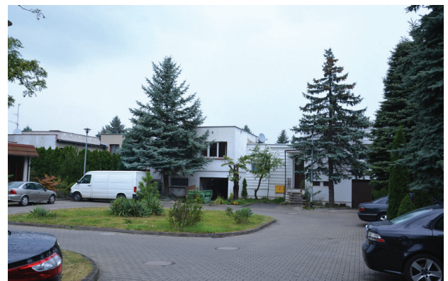
Fig. 11. The colony of patio houses Youth Estate, designed by L. Konarzewski, Wrocław.
