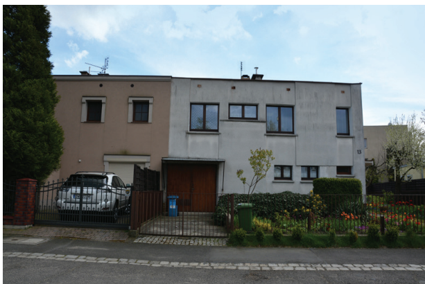
Fig. 3. Semi detached house of Budowlani housing estate, designed by W. Molicki, R. Spławski. An example of thermal modernization (left side), the original windows design on the facade has been changed. Stylized window bands were introduced (photo by Z. Napieralska)
