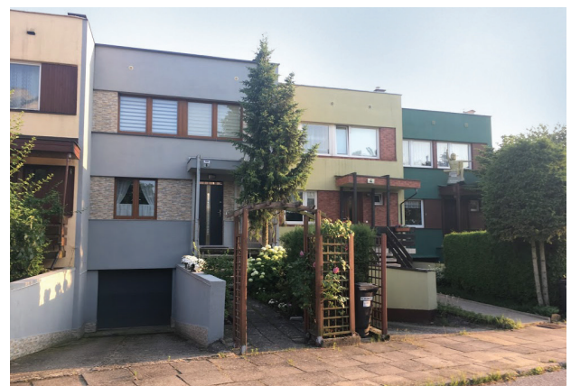
Fig. 7. Wspólny Dom detached house settlement in Szczecin city, the current state of the buildings after modernizations. Originally designed wooden panels have been changed with different materials: stone mosaic, brick tiles or justifies by different color (photo by Z. Napieralska)
