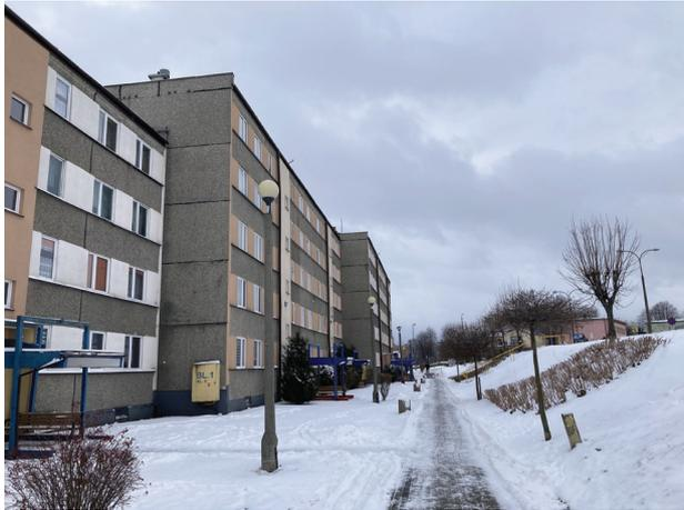
Fig. 1. View of one of the buildings. The thermal modernization so far has been limited to thermal insulation of window strips. The difference in the ground level is also visible (photo by R. Oleksik)
