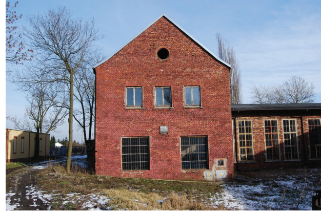
Fig. 6. Workshop and social building (photo by P. Mierosławski)
