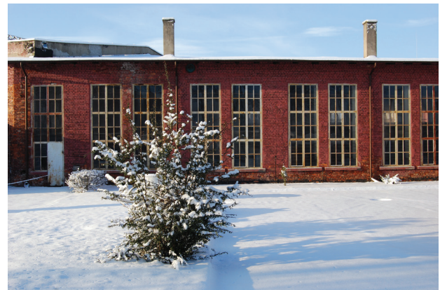
Fig. 7. View of the machine hall (photo by P. Mierosławski)
