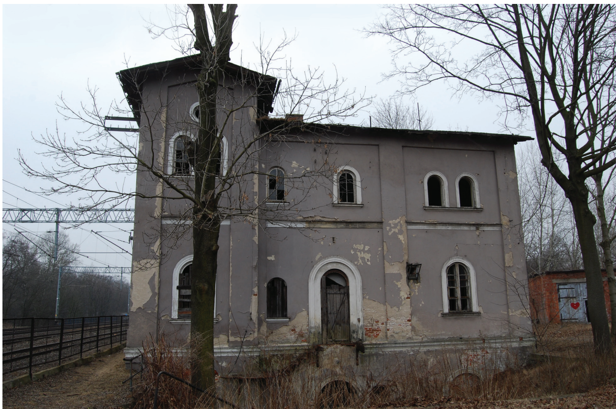
Fig. 3. Former water tower (photo by P. Mierosławski)
