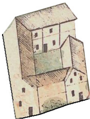
Fig. 4. Wrocław, Old Town, 17 Mennicza St., medieval malt house (according to the Weihners' plan)
