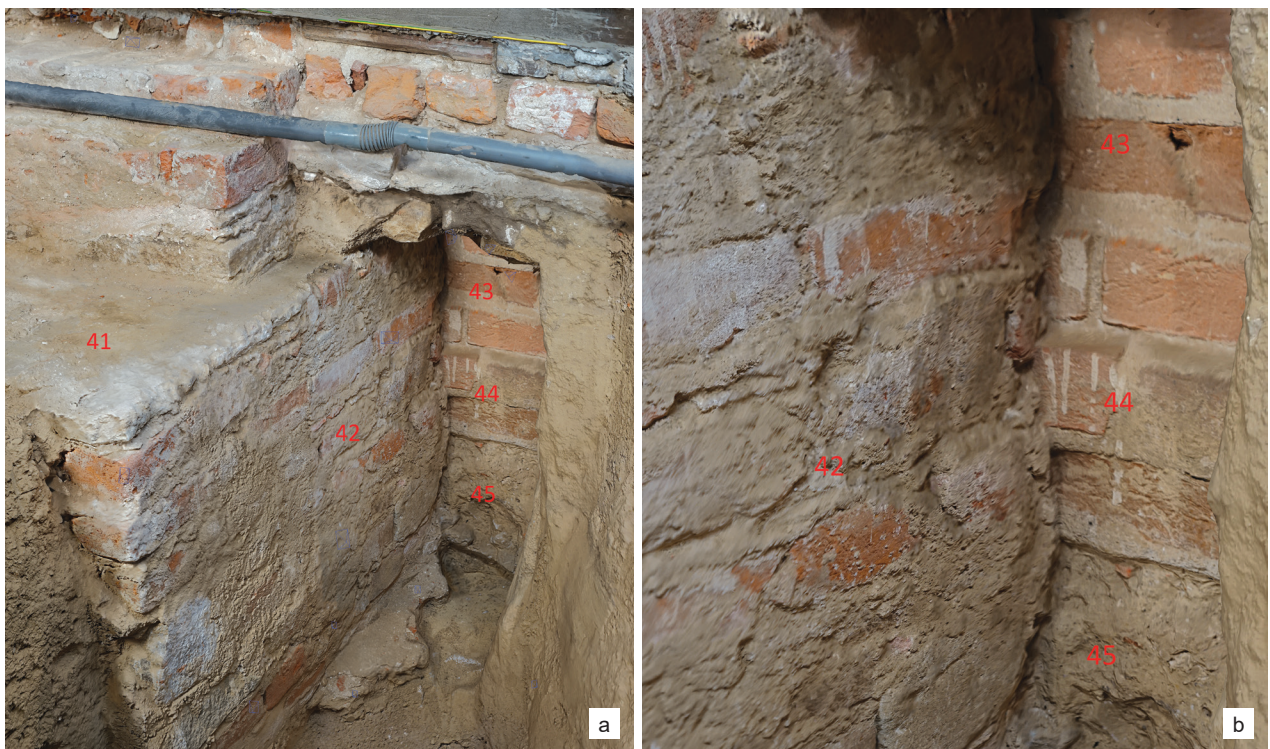
Fig. 7. Sandomierz, Church of St. James, east section of the excavation (SW-side view): a) relation between constructions k. 41/42 (newer, appended), b) k. 43/44 (older) (elaborated by A. Gołębnik)
