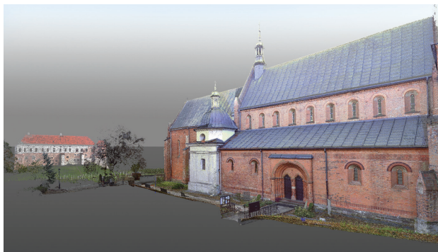
Fig. 1. The orthophotogrammetric projection – Church of St. James in Sandomierz – displaying the northern elevation (elaborated by A. Gołębniak)
