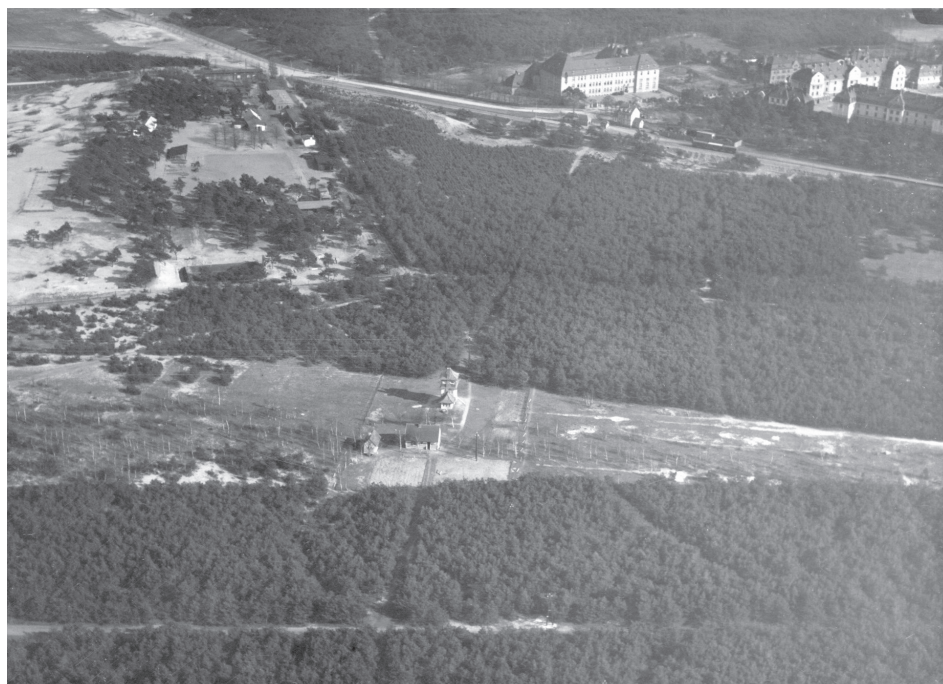
Fig. 8. Toruń – aerial photo with the Nowe Bielany pumping station visible (1933) (source: APT, AmT D, ref. no. 1648)
