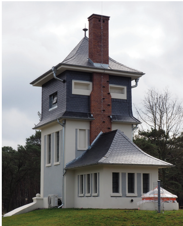
Fig. 3. Toruń – the former Nowe Bielany pumping station: machine room building (photo by D. Jagiełło, 2024)
