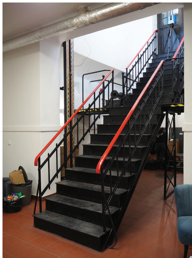
Fig. 6. Toruń – the former Nowe Bielany pumping station: stairs leading from the pump hall to the ground floor of the machine room building (photo by D. Jagiełło, 2024)
