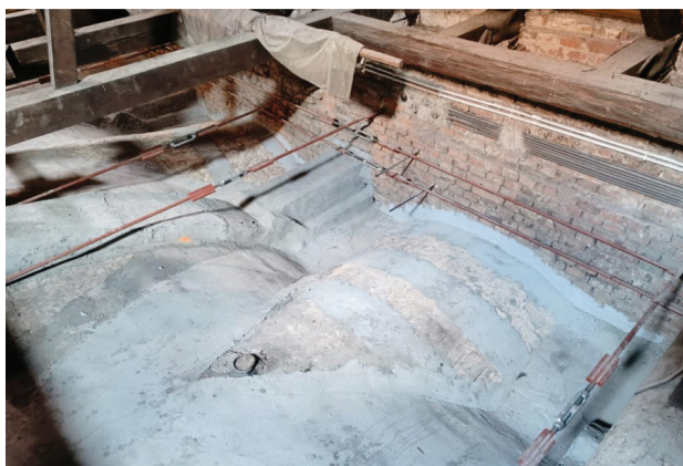
Fig. 4. Vault after reinforcement (photo by Ł. Bednarz)
