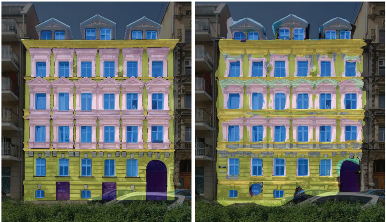
Fig. 3. Ground truth annotation and semantic segmentation results on the NeoFaçade dataset (elaborated by D. Hardzetski)
