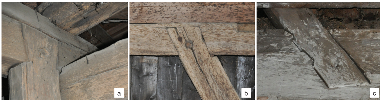
Fig. 9. Church of Our Lady of the Rosary in Byków, list of carpentry joints – lap joints: a) double dovetail lap joint-shaped, b) single dovetail lap joint-shaped, c) double-notched (photo by U. Schaaf, 2022)
