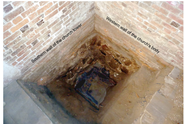
Fig. 7. Toruń, St. James's Church from the interior. Uniform foundation of the tower and western wall. Bird's eye view (photo by B. Kriks)
