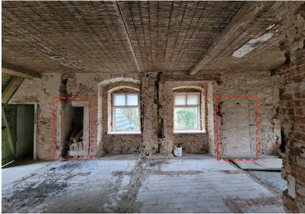
Fig. 9. Stöckel Palace, preserved remains of two latticework bays together with the battered frame of the passage through the east gable wall (photo by A. Walkowska)
