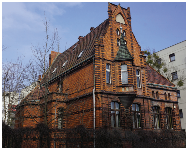
Fig. 4. Toruń, villa at 84 Krasieński Street, built in 1899 (photo by D. Bręczewska-Kulesza)
