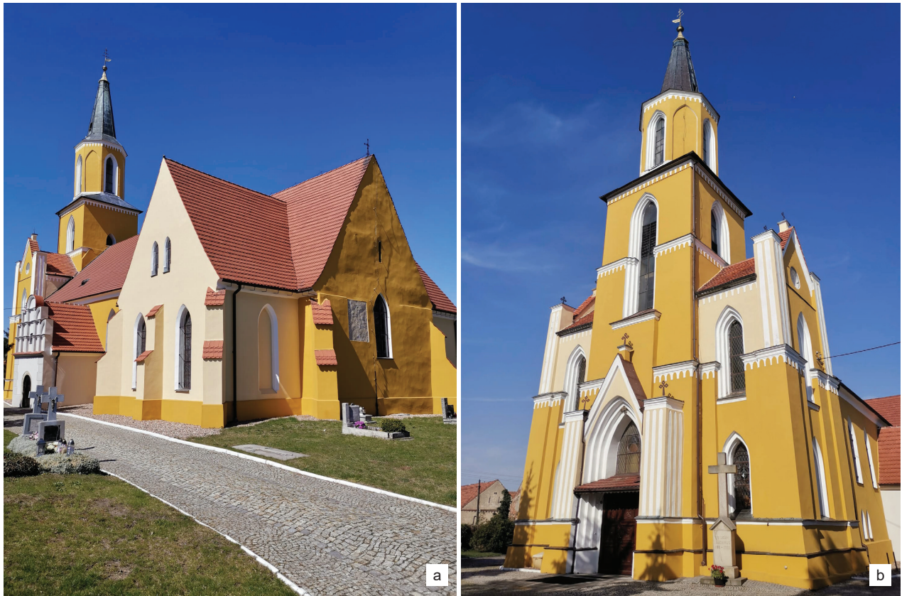
Fig. 3. The church in Kostomłoty after renovation of the façade in 2024: a) view from the west, b) view from the front (photo by R. Kupczak, 2024)
