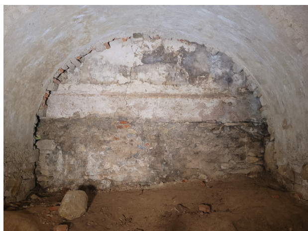
Fig. 3. South wall of part B of the crypt containing plasterwork from the medieval period and three different floor levels, 2023 (photo by A. Piwek)
