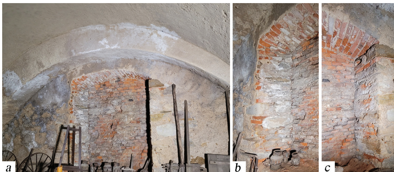
Fig. 2. South wall of part A of the crypt with two arches (wall and added) and a bricked-up exit to the monastery grounds, 2023: a) general view, b) eastern glyph, c) western glyph (photo by A. Piwek)
