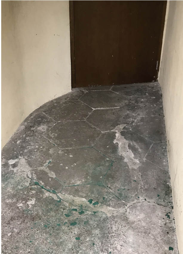
Fig. 5. Outline of the semicircular staircase (also marked by the curvature of the south wall) in the passageway of the eastern wing of the monastery leading to the added pavilion, 2023 (photo by M. Kwasek)
