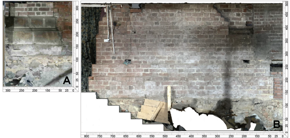
Fig. 3. Foundations of the pillars of St Elizabeth's Church in Wrocław: A – nave, B – chancel (orthophotos generated on the basis of a photogrammetric model; elaborated by F. Hackemer)
