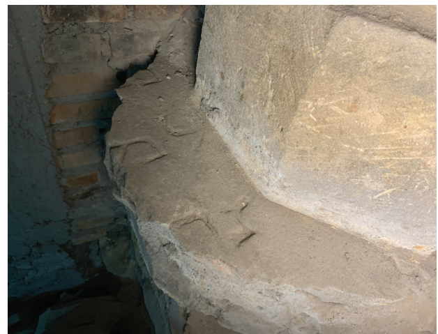
Fig. 7. Fraction of a matzeva used as a floor slab under the fifth pillar from the west in the north aisle (elaborated by F. Hackemer)
