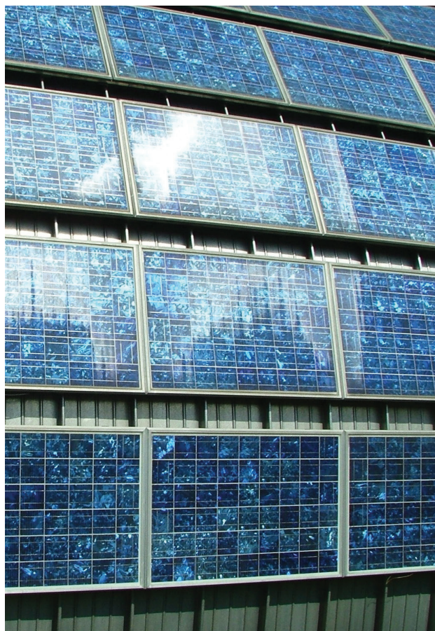
Fig. 2. Scheuten Solar, Gelsenkirchen (1999). PV modules with a visible crystalline cell structure and a regular grid pattern, mounted on standing seam aluminium cladding (photo by M. Muszyńska-Łanowy)
