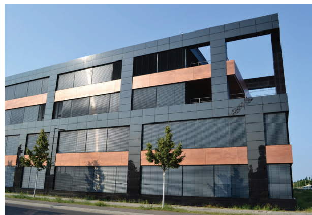
Fig. 3. Solteature facility, Berlin-Adlershof (2009). Black thin-film CIS modules form a sleek, monolithic surface with strong architectural coherence (photo by M. Muszyńska-Łanowy)
