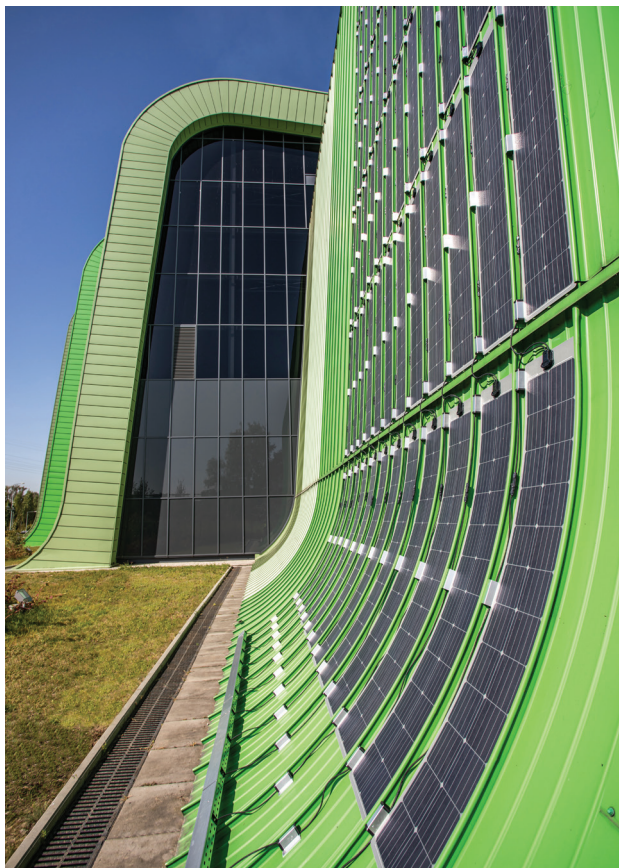
Fig. 5. Eco-incinerator, Kraków (2019). Flexible m-Si PV modules following the curved geometry of the green metal façade; the exposed and rhythmically repeated layout emphasizes the expressive character of the industrial building (source: courtesy of KHK SA Archives)
