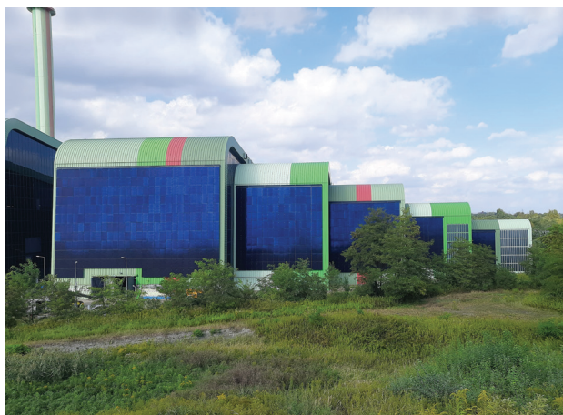
Fig. 6. Eco-incinerator, Kraków (2019). Two different PV technologies on the building façades. The vivid blue of the rigid glass BAPV creates a striking visual effect against the original envelope (source: courtesy of KHK SA Archives)
