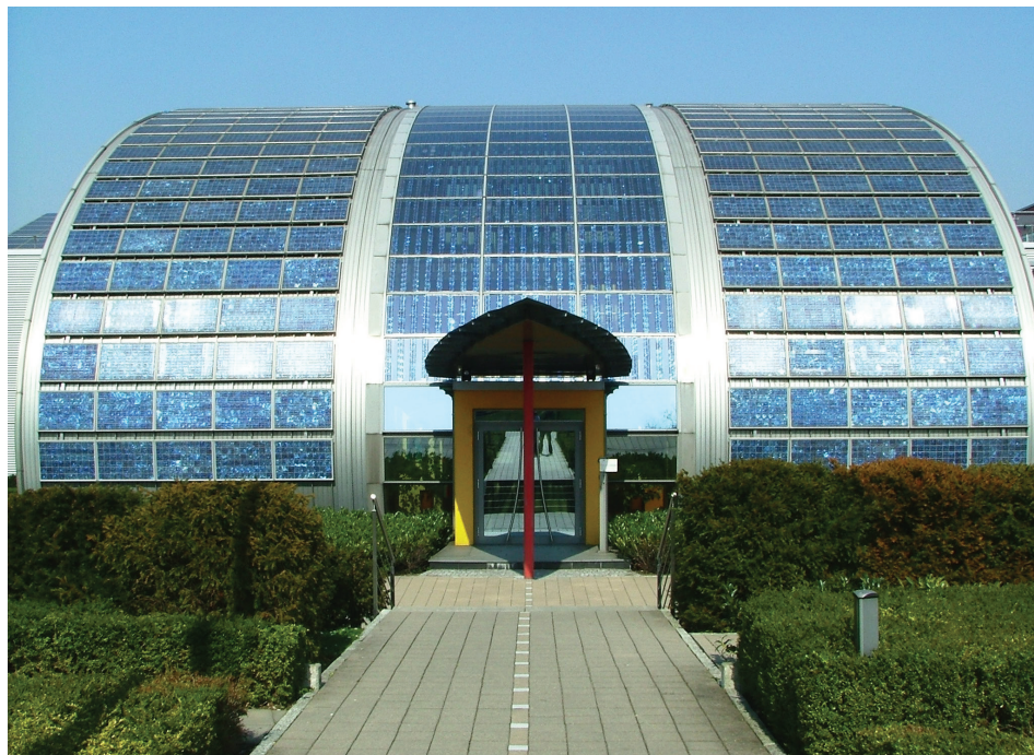
Fig. 1. Scheuten Solar, Gelsenkirchen (1999). A pioneering example of PV integration in an industrial building façade (photo by M. Muszyńska-Łanowy)
