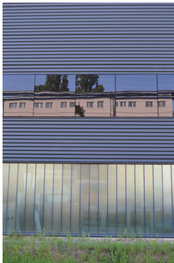
Fig. 4. Solteature, Berlin-Adlershof (2009). BIPV CIS modules with a reflective surface, seamlessly aligned with the corrugated metal cladding; the dark, mirror-like finish visually conceals the solar function (photo by M. Muszyńska-Łanowy)
