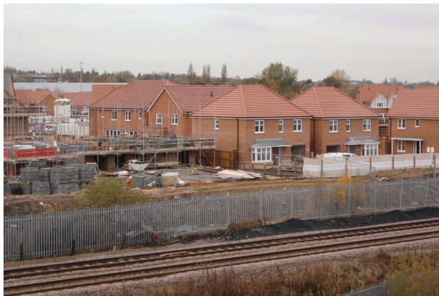
Fig. 4. Redeveloped Prince of Wales Colliery, Pontefract, England (photo by Derek Dye, source: www.geograph.org.uk/p/5652321 , CC-BY-SA/2.0; accessed: September 5, 2026)
