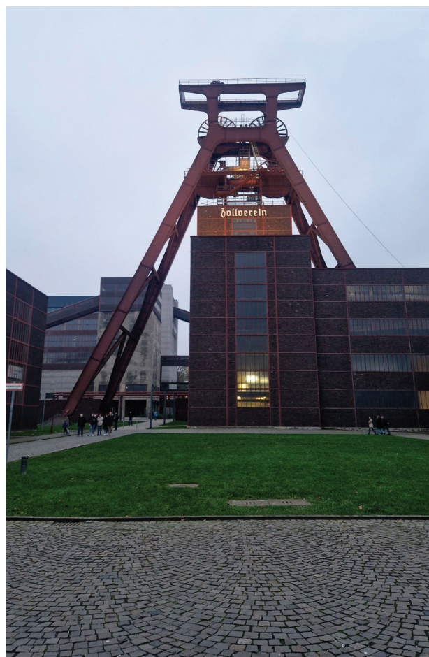
Fig. 2. Redeveloped Zollverein mine in Essen, Germany (photo by K. Pieter)
